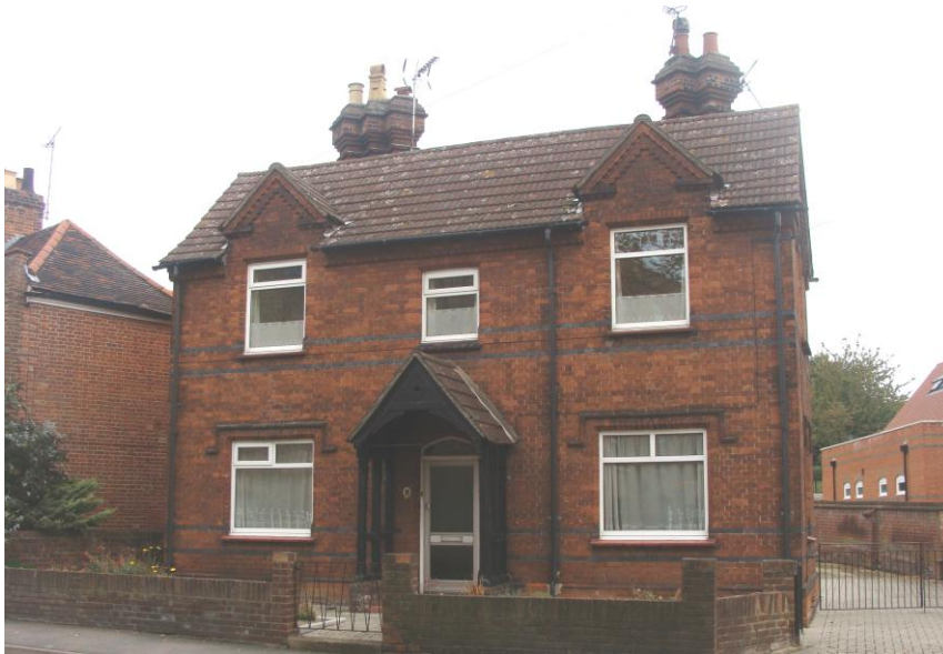
Picture 29 – 19 th century building of pleasing mass and proportion has been compromised by modern windows that are unsympathetic.
