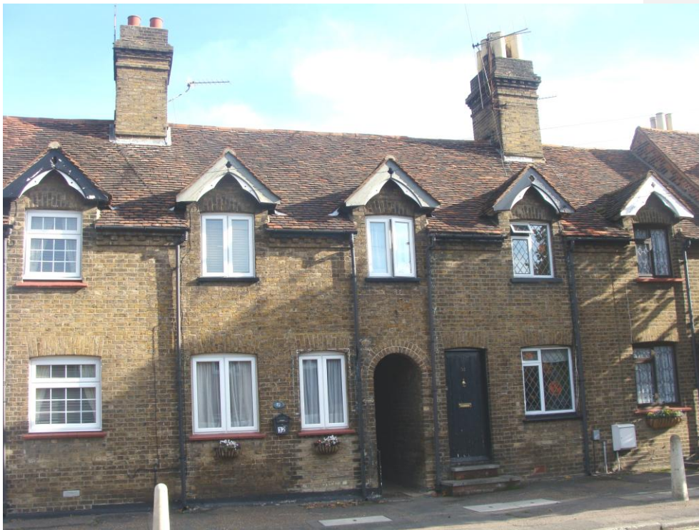
Picture 21 - Nos. 32 - 34 Roydon Road. Their attractive general mass and repetitive historic architectural detailing is compromised by a common problem in the village, namely one of modern windows of uncoordinated and often unsympathetic design.
