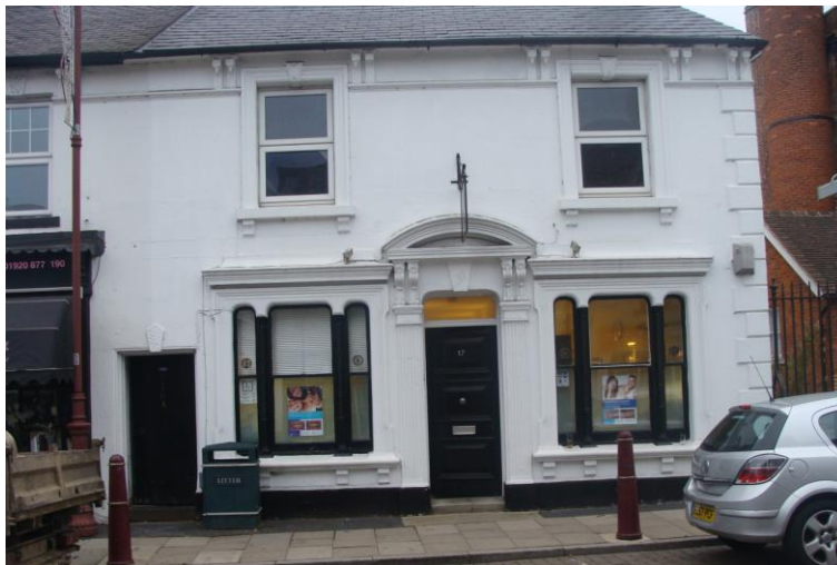
Picture 8 – Good quality shop front retained and sympathetically painted without brash colouring or detracting advertisements.
