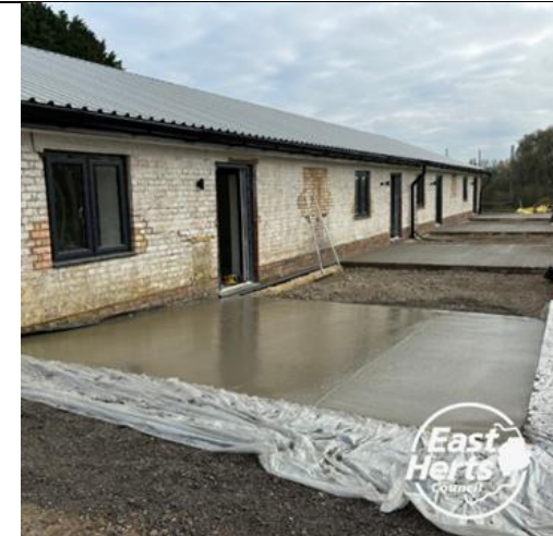
Figure 14 works in progress at Skill at Arms
