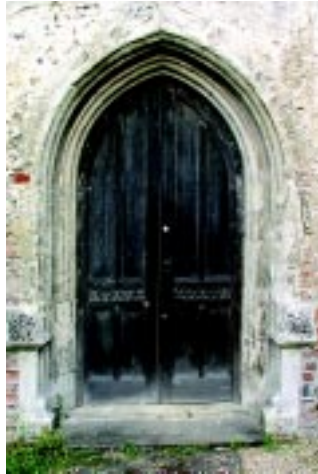
The Bell Tower door
