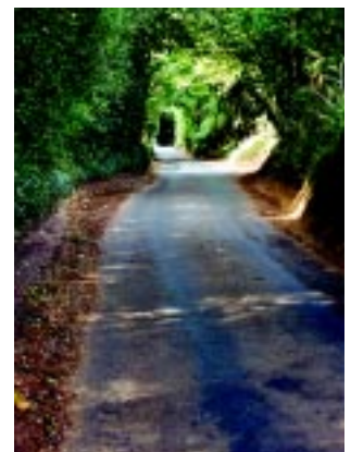
An eroded Lanterns Lane, today
