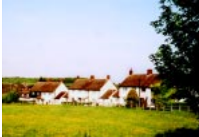
Stringers Lane from Centre Field
